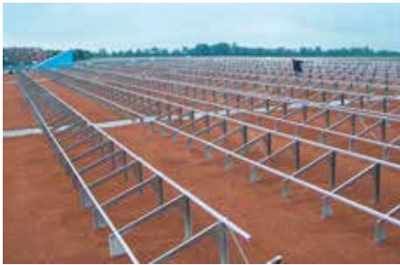
4. The Solar Bases are covered with system substrate as per the required load.
