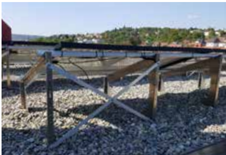
Two pre-punched flat aluminium profiles for crosswise stabilization of two Solar Base Frames.
