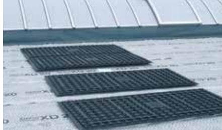
2. The Solar Bases SB 200 are laid over the Fixodrain® XD 20.
