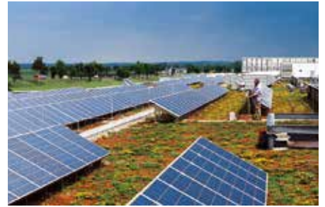
6. Roof with fully-installed solar energy system.
