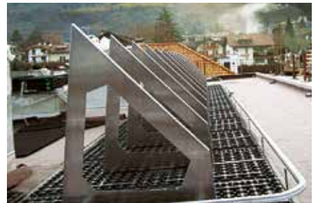
Frame 45° for solar thermal panels on a roof area with a 5° slope.
