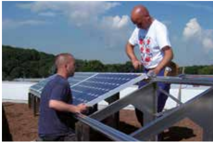
5. The solar panels are installed.
